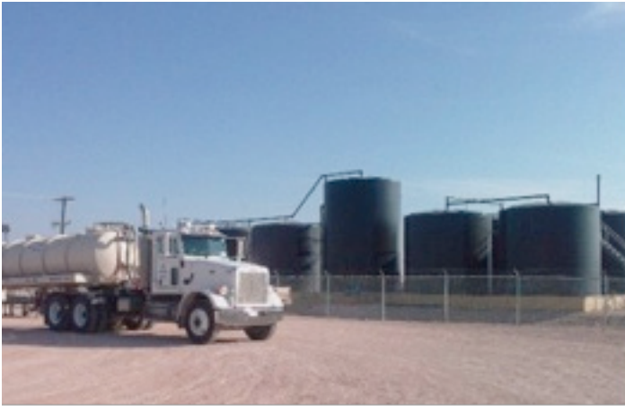
Truck unloading into tank battery for saltwater/oil storage and separation
