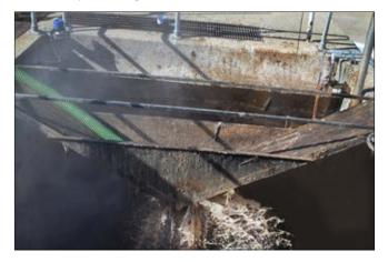
An Echotel<sup>®</sup> ultrasonic transmitter from Magnetrol measures grease level through a fog of vapor at the WWTP grease receiving station. Grease is being fed from a tanker through the green hose.
