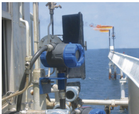
Due to environmental laws and restrictions, oil and gas platform operators must monitor and report the amount of flared gases. The consistent composition, low flow sensitivity, and high turndown capabilities make the TA2 an ideal flow meter for this service.
